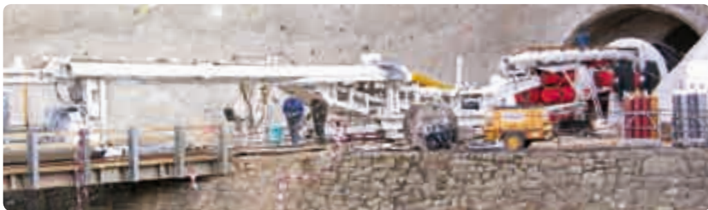
Construction of gallery with tunnel boring machine
