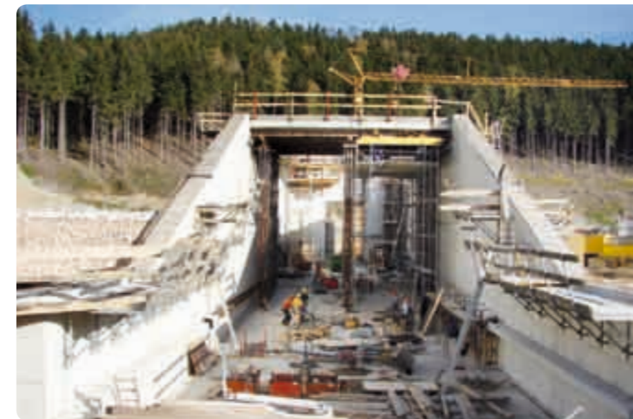
Construction of pre-dam
