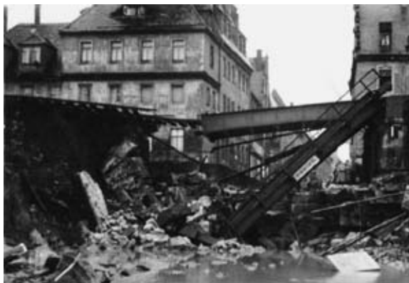
Fig. 15: Town of Pirna after the river Gottleuba flooded in 1957 (photo: LTV)
