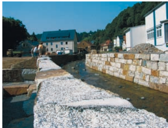
Fig. 20: Same revetment of the Müglitz stream in Glashütte, 2004 (photo: LTV, 2004)
