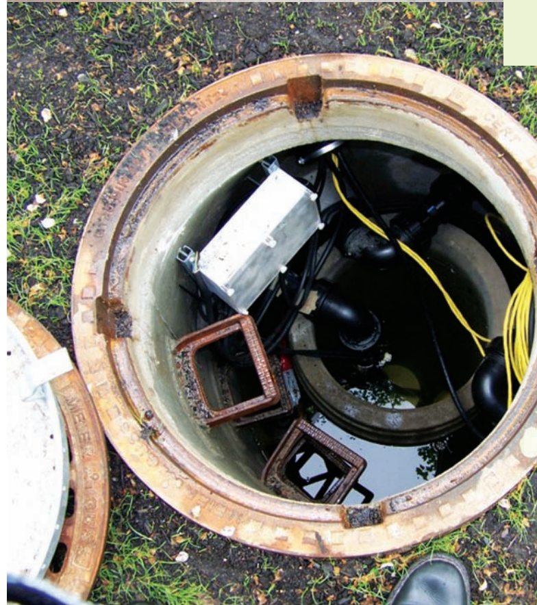
Manhole with entry point to the sewage pipe
