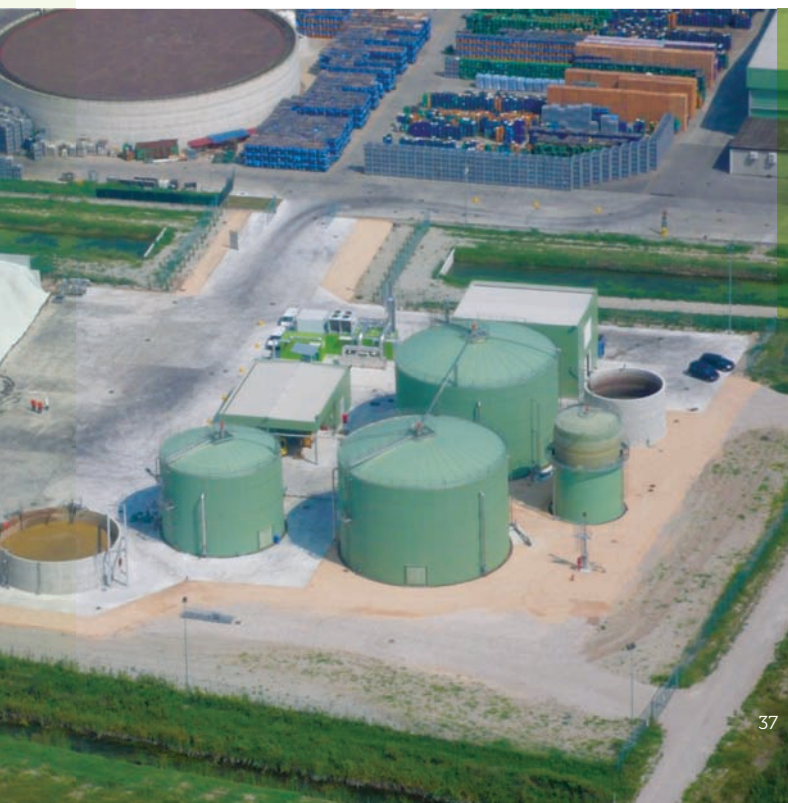
Biomass cogeneration plant
