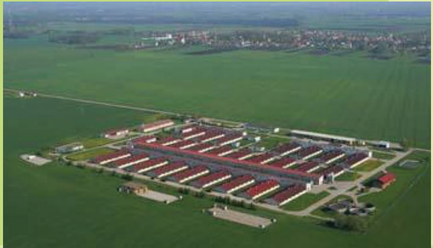
Aerial view of biogas plant in Żerniki Wielkie
