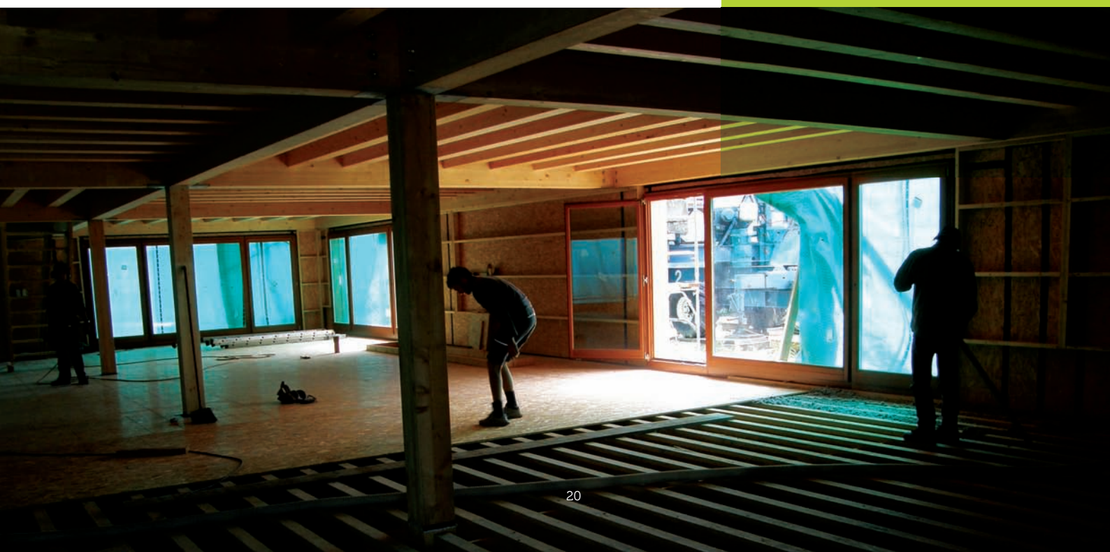
Wooden roof structure of the Energy Advice Centre
