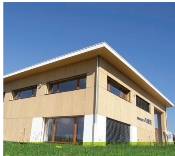
Energy Advice Centre in Meythet
