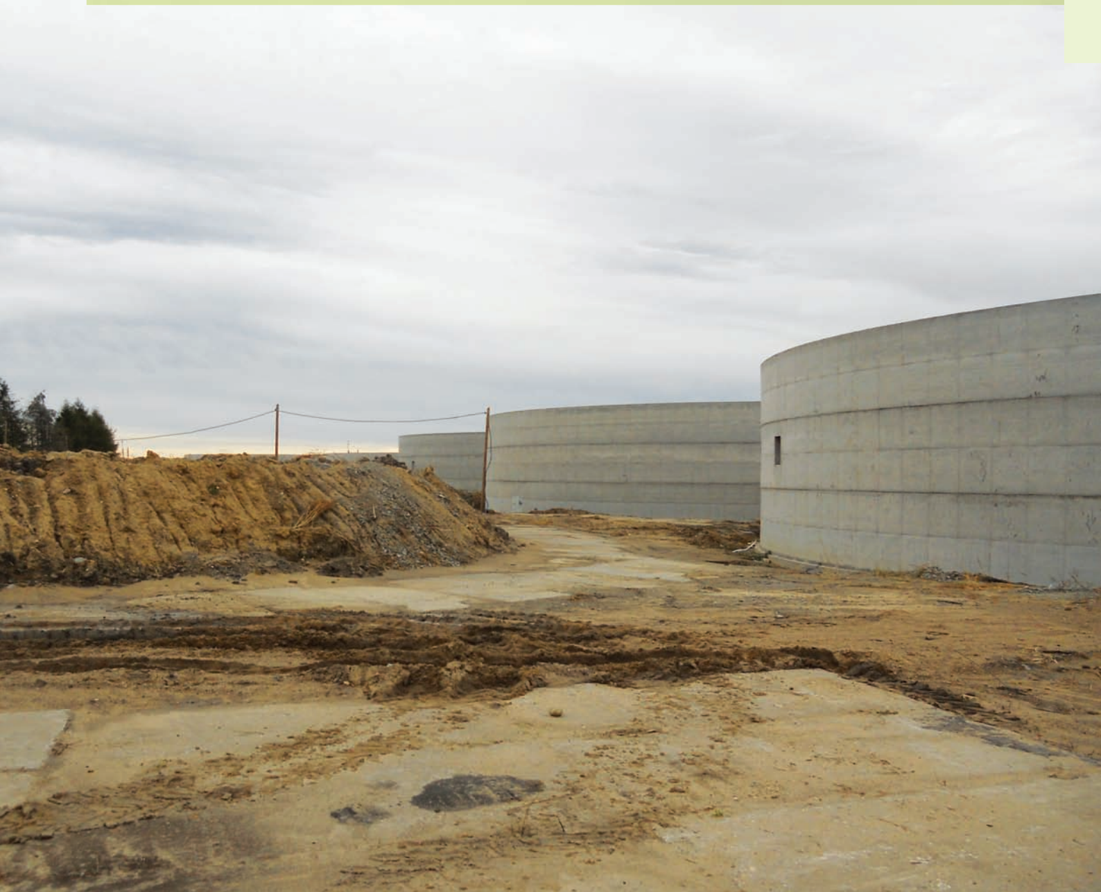
Biogas plant construction is nearing completion
