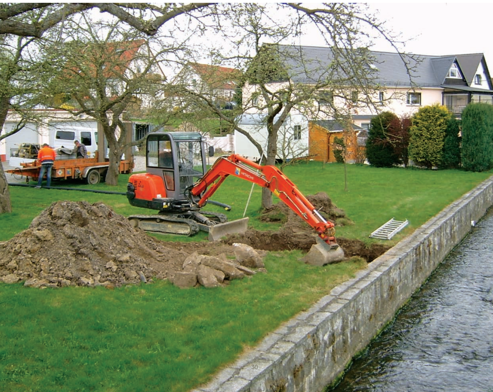
Construction works at Haselbach River
