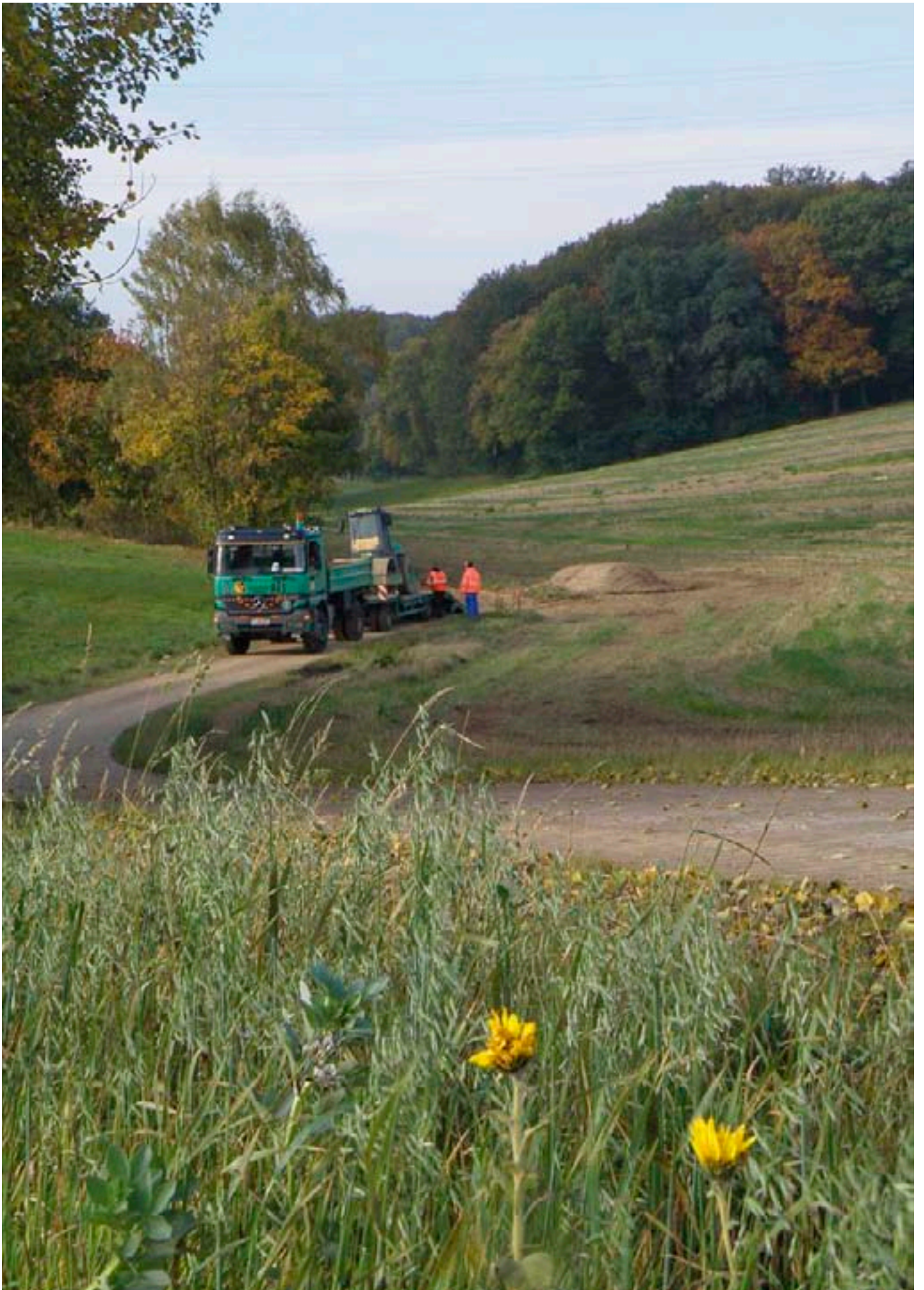
Construction of a rural on Schönberg farmland
