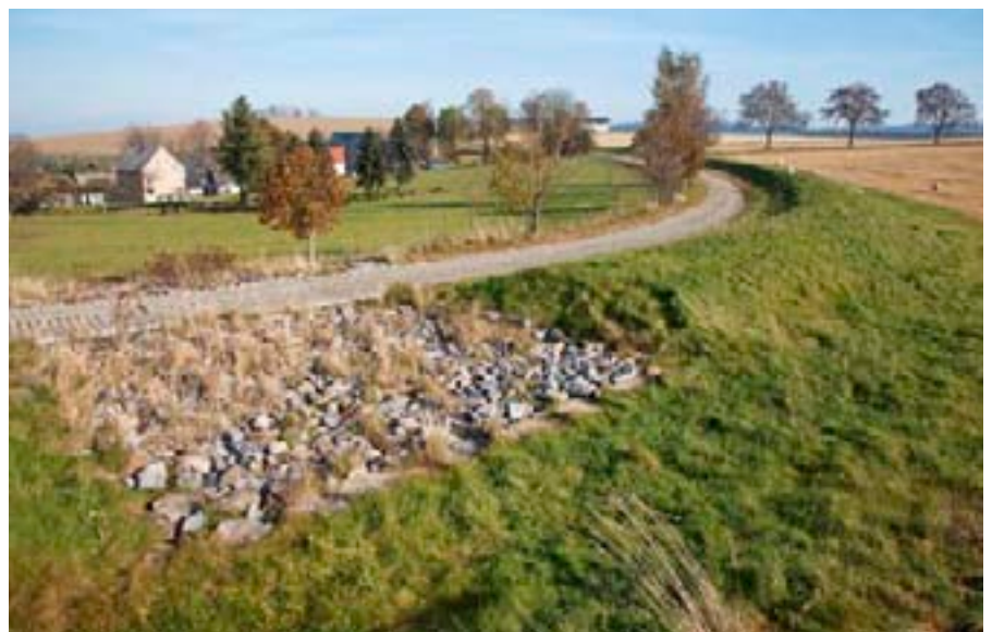
Completed flood control dam with spillway and farm road – catchment area A1. The locale to be protected is seen in the background.
