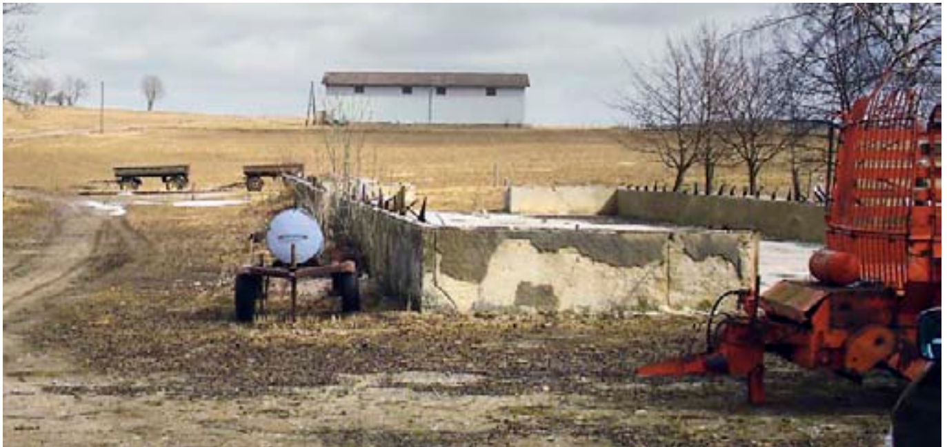
Remains of the former machine hall; photo: Dittersbach Community of Participants
