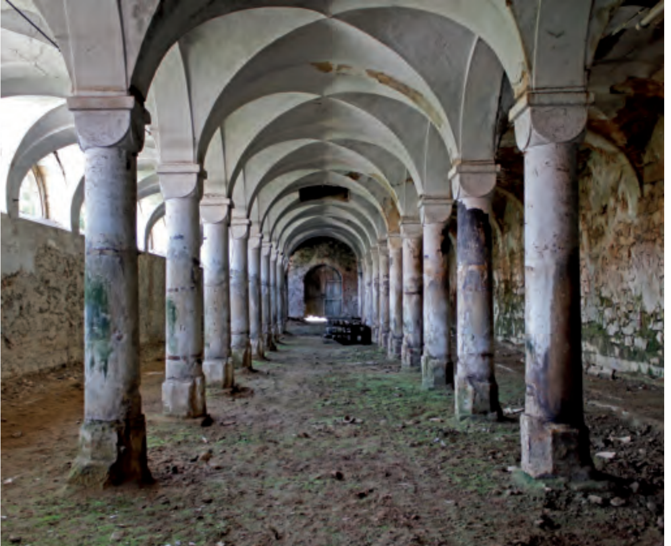
Interior view of the three rowed stables
