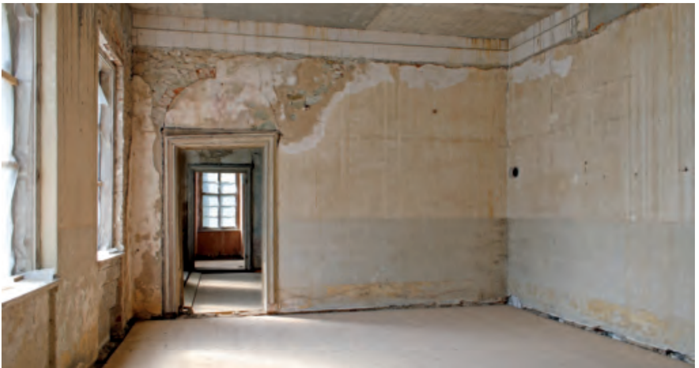
View of one of the rooms
