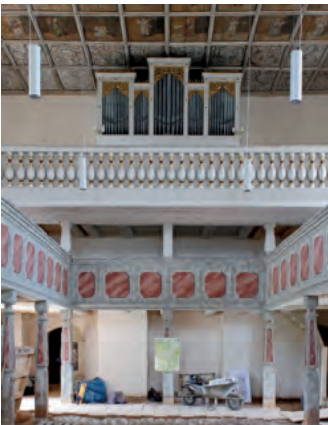
View of the organ gallery during construction work
