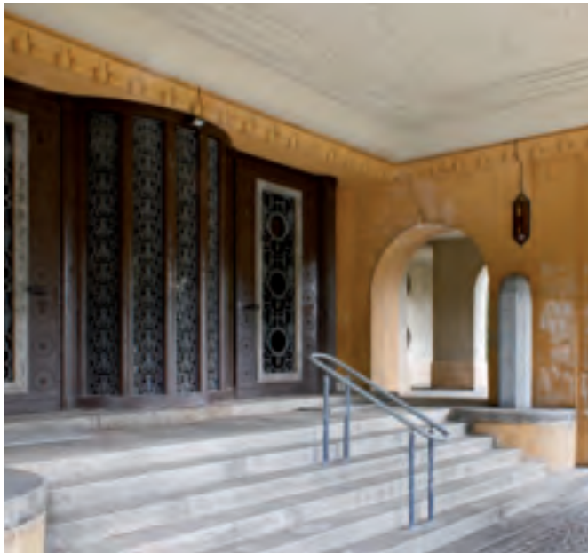
Portal situation at the front of the tower
