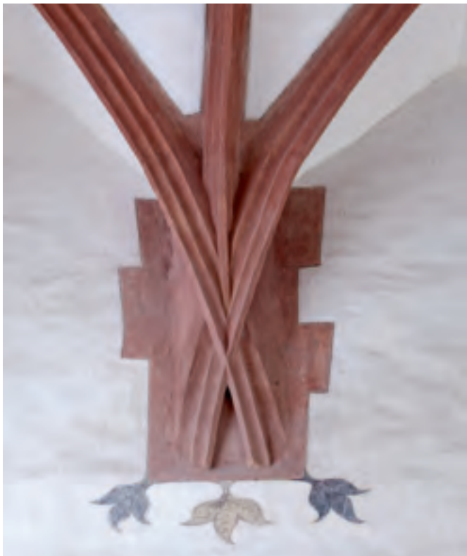
Start of the vaulting in its original form
