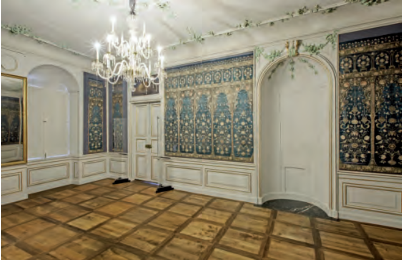
Section of the wall after the restoration with an alcove for an oven
