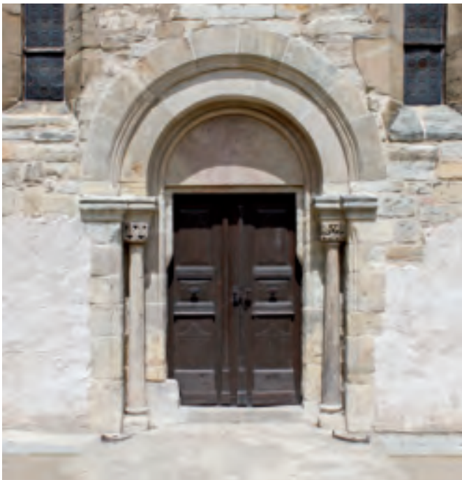
Portal at the southern transept
