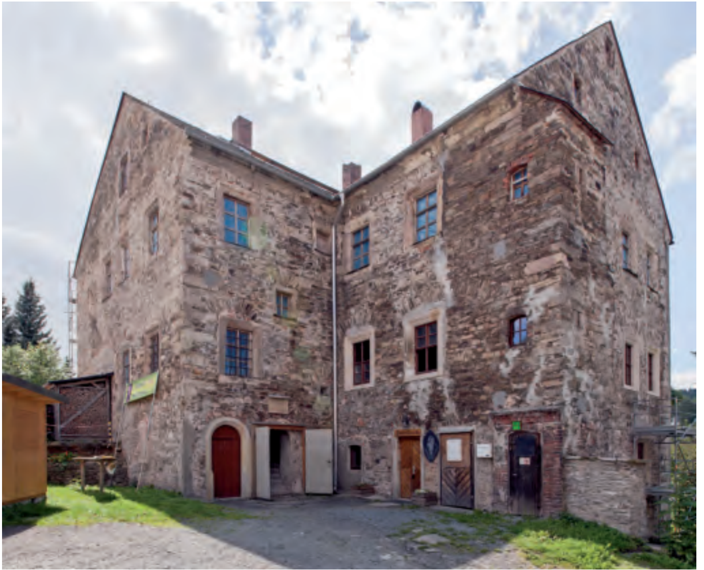
Exterior view with entrance portal
