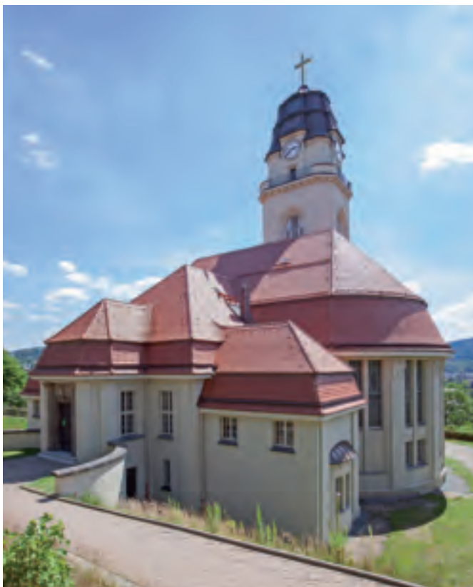
View from the hillside with roof valleys with beavertail roofing
