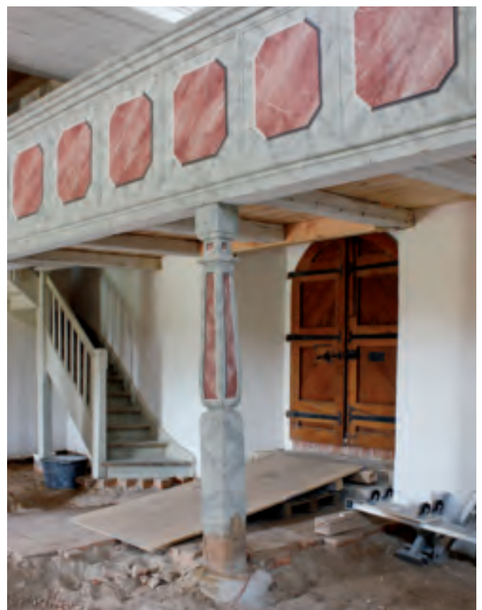
Gallery with original colours after the floor covering was removed
