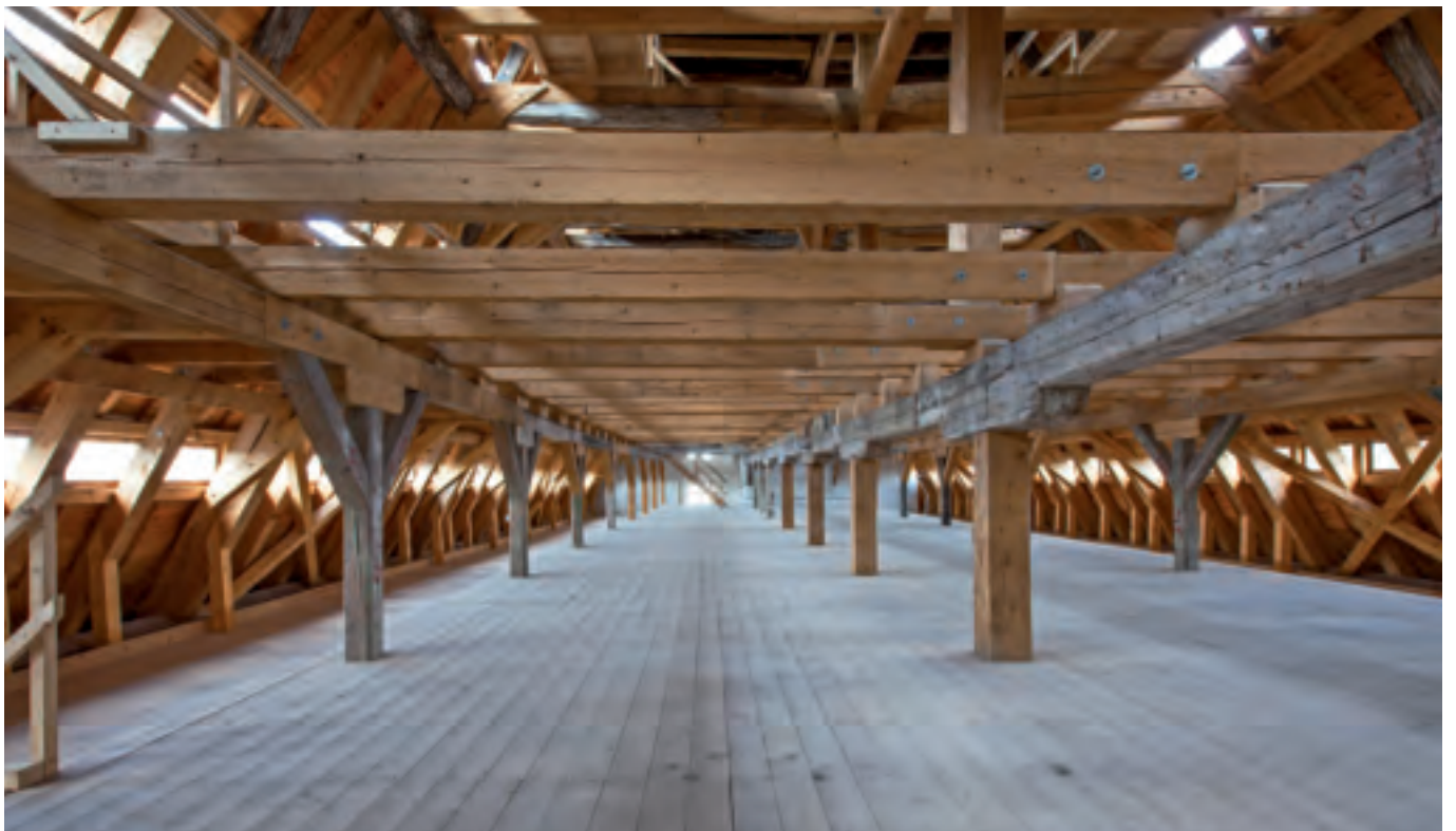
View into the roof truss
