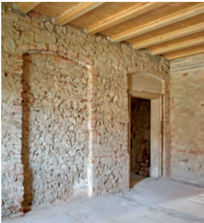
Foyer with completed wooden beam ceiling
