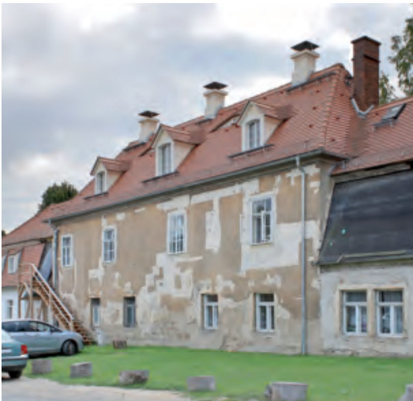
New roofing and test exposures on the street façade
