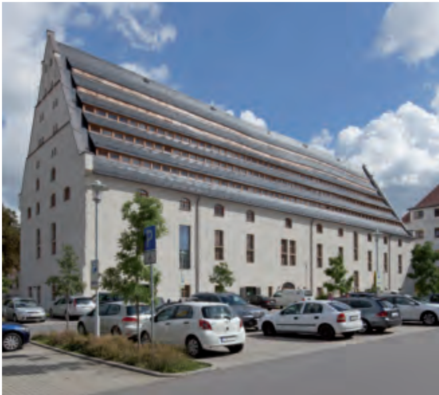
View from the southwest
