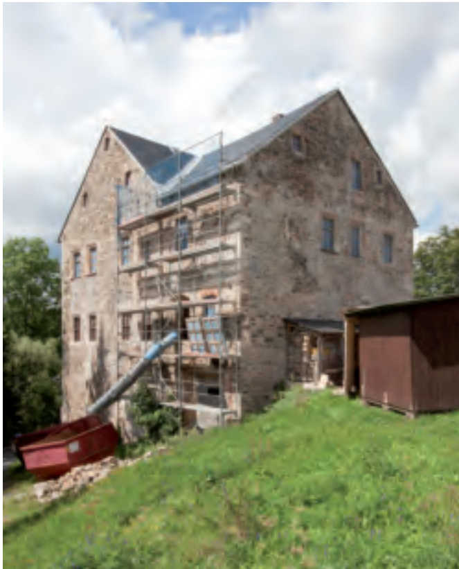
View from the southeast
