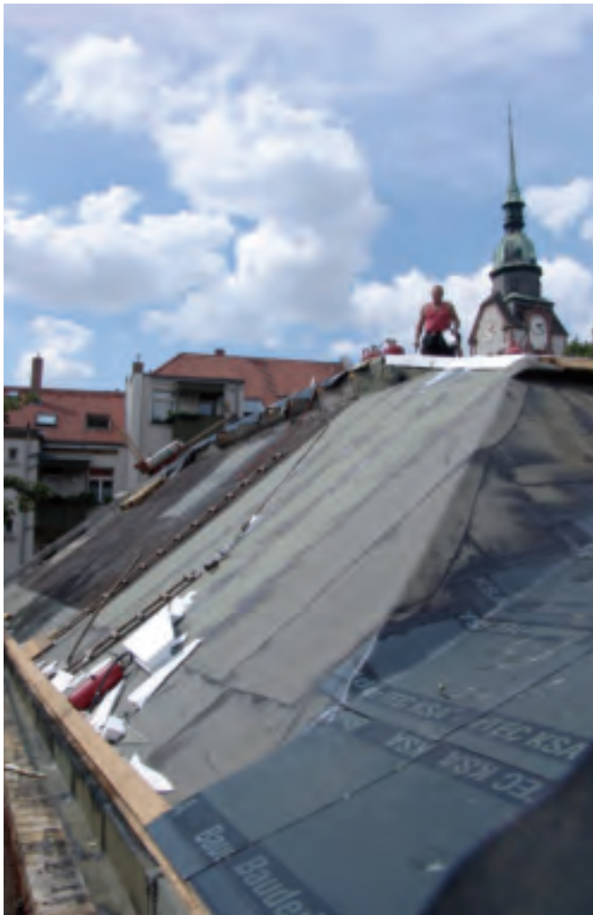
Roof during the re-roofing in 2006
