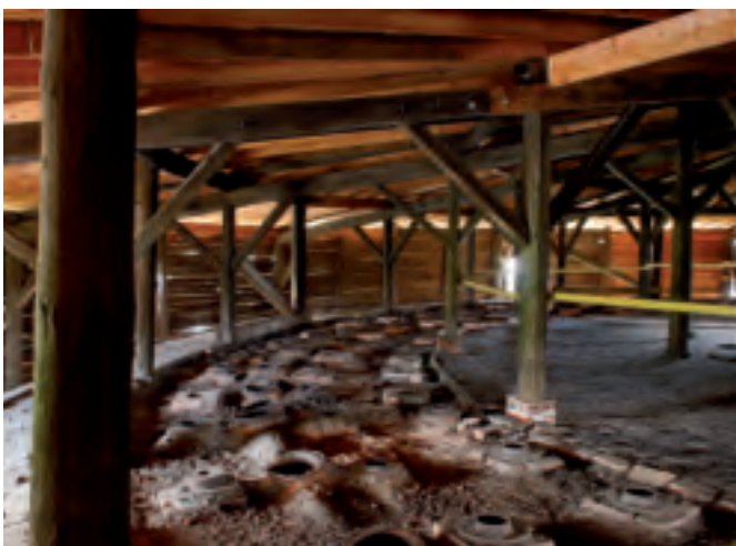
Drying loft with repaired roof
