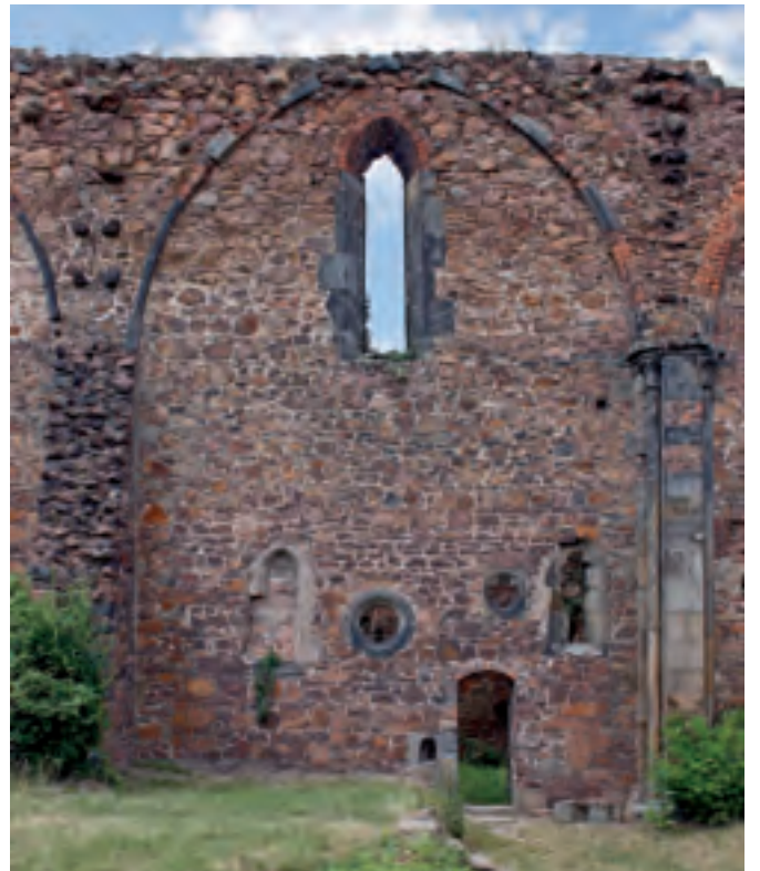
View of the demolition edge of the former vaults
