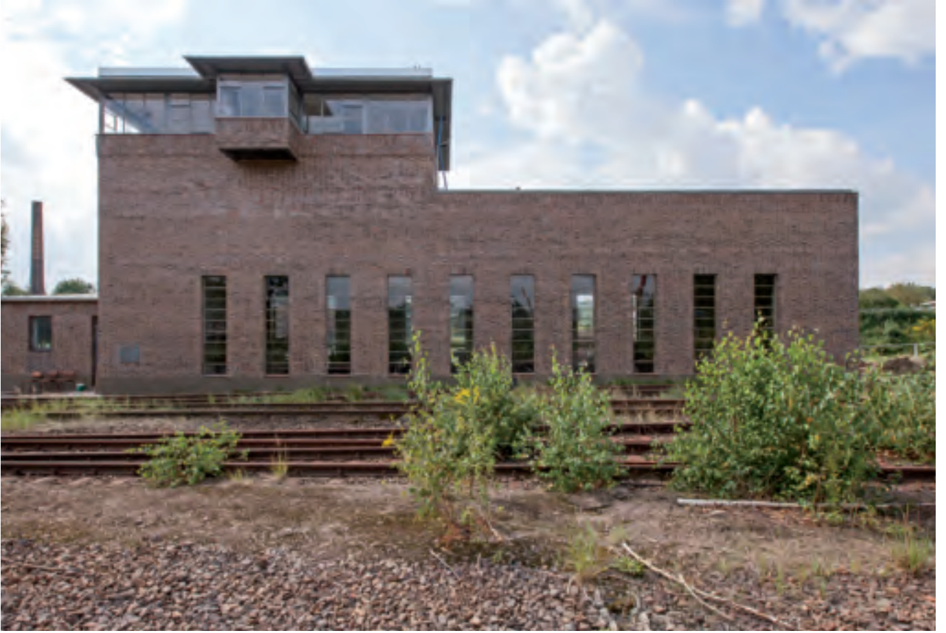
Machine house of the cable system with mounted switch tower 2
