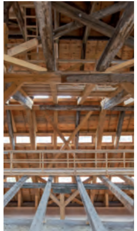
Roof truss after strengthening
