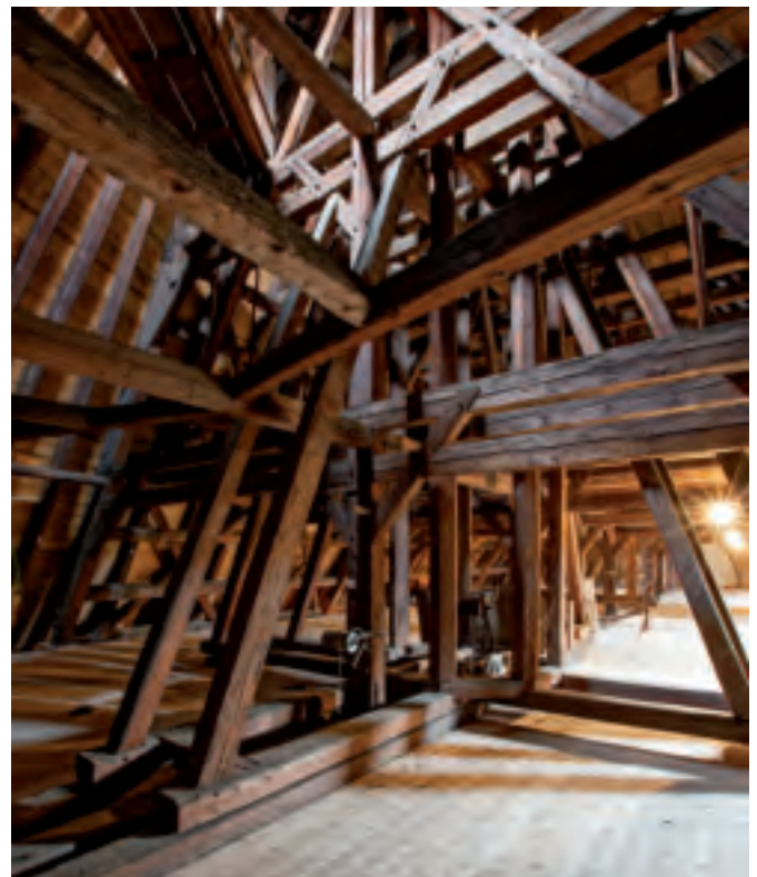
Wooden roof construction
