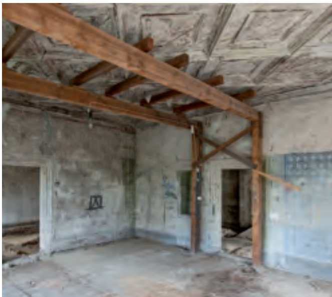
Panelled ceiling on the first floor
