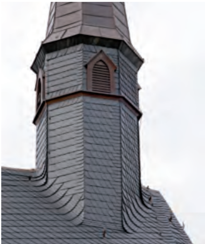
Ridge turret with a natural slate covering
