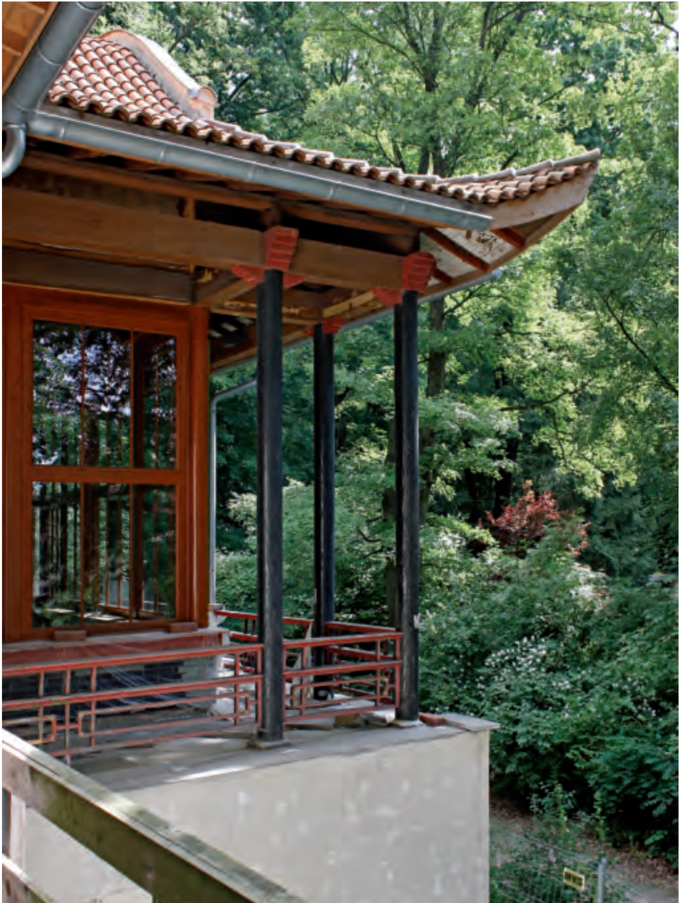
Detail during renovation
