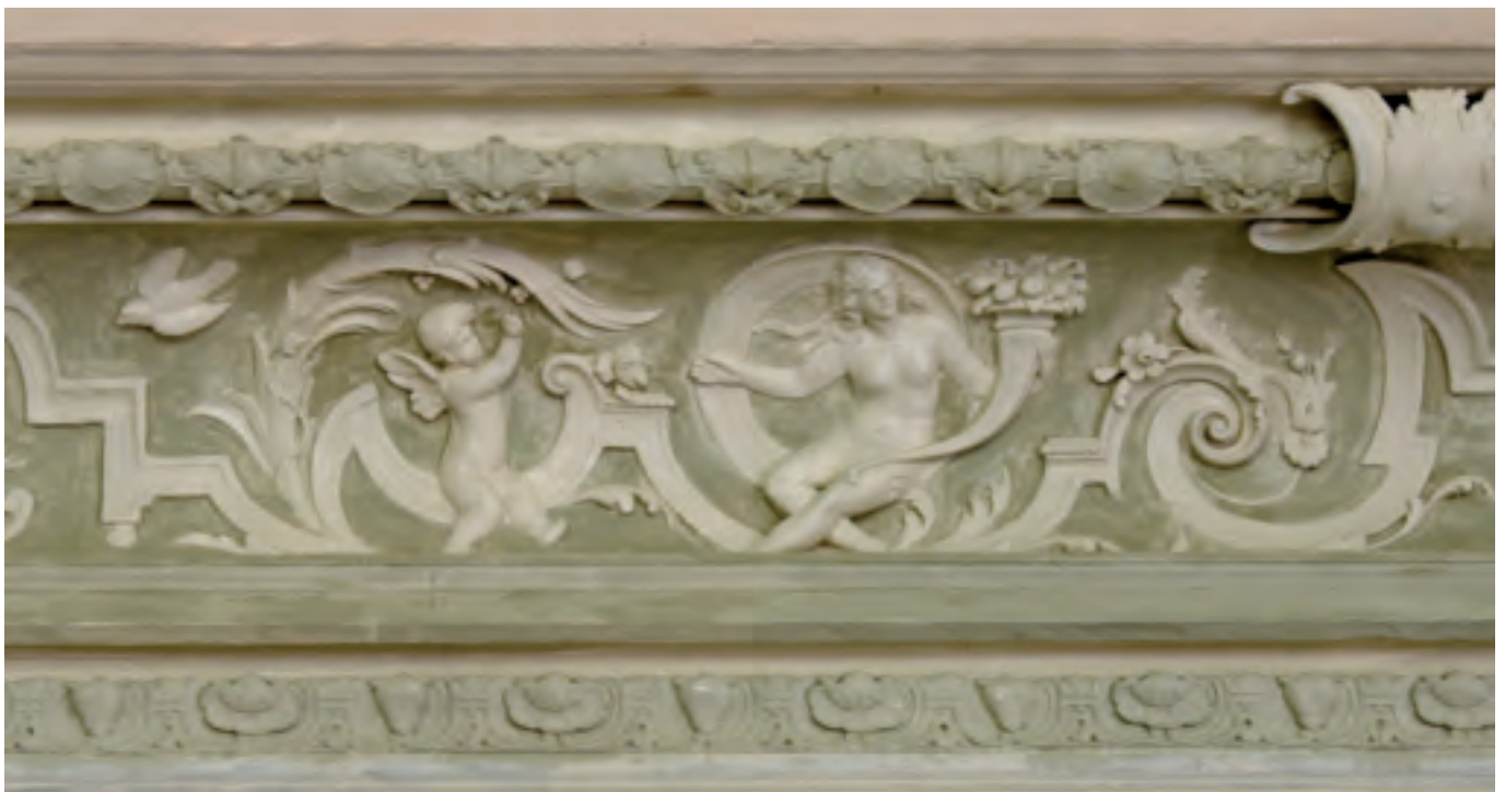
Detail of a hollow stucco moulding
