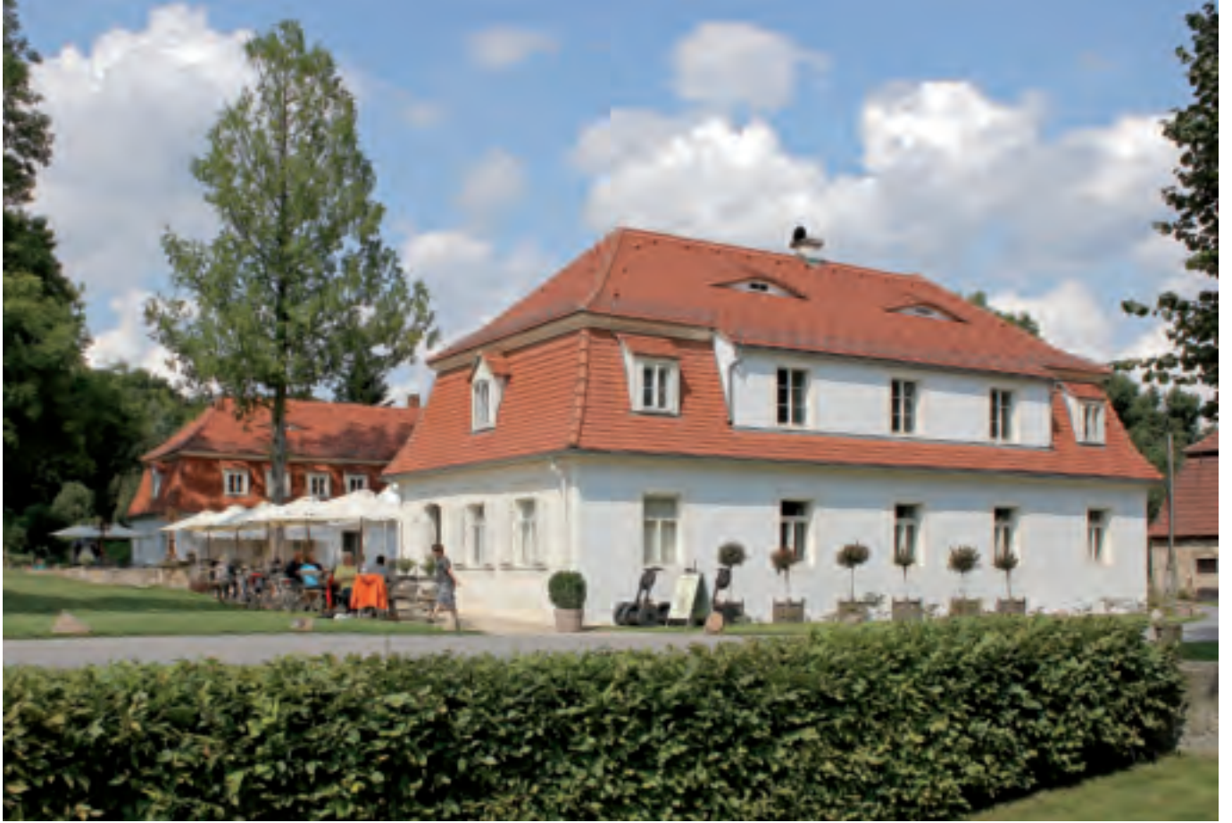
View from the yard
