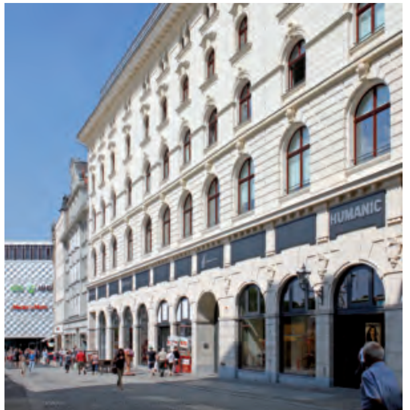
Façade facing Hainstraße
