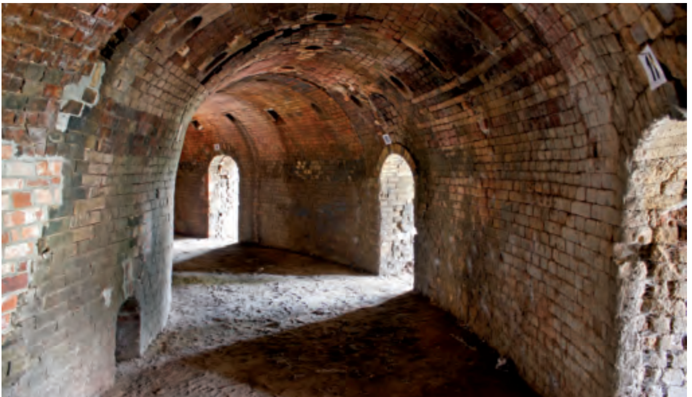
View into the ring-shaped kiln
