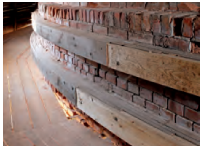
Repaired perimeter of the kiln
