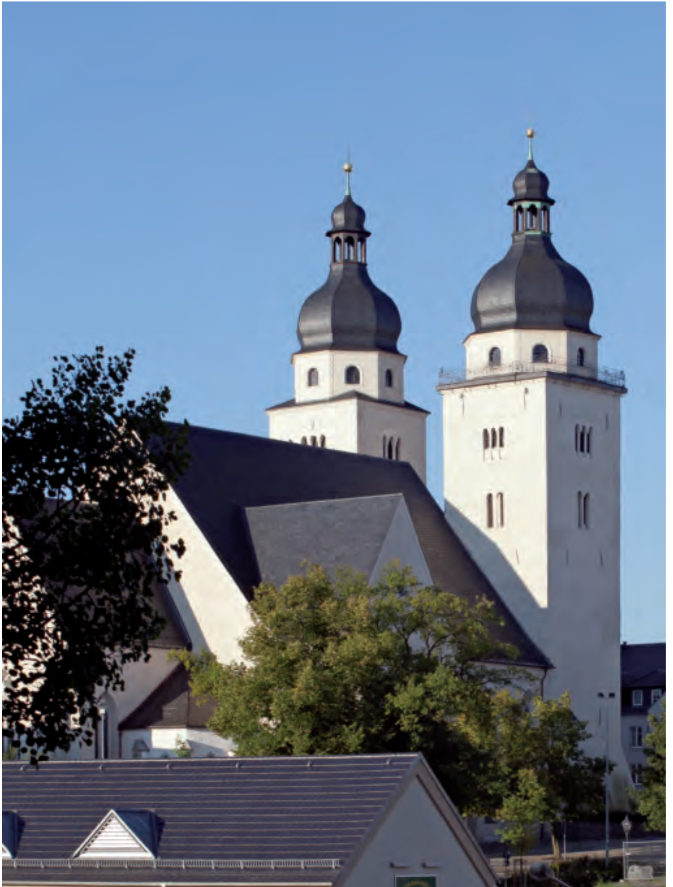
View from the northeast, looking at the nave and double towers
