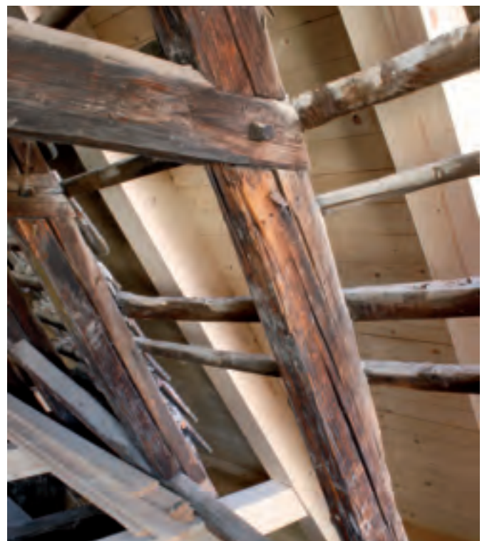
Late gothic roof construction with new roof over top, detail
