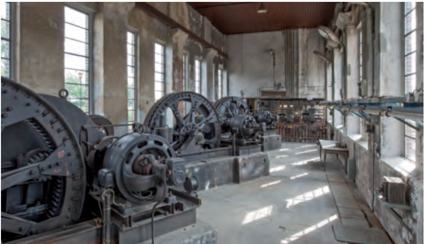
View of the inside of the machine house with the three drive units of the endless cables
