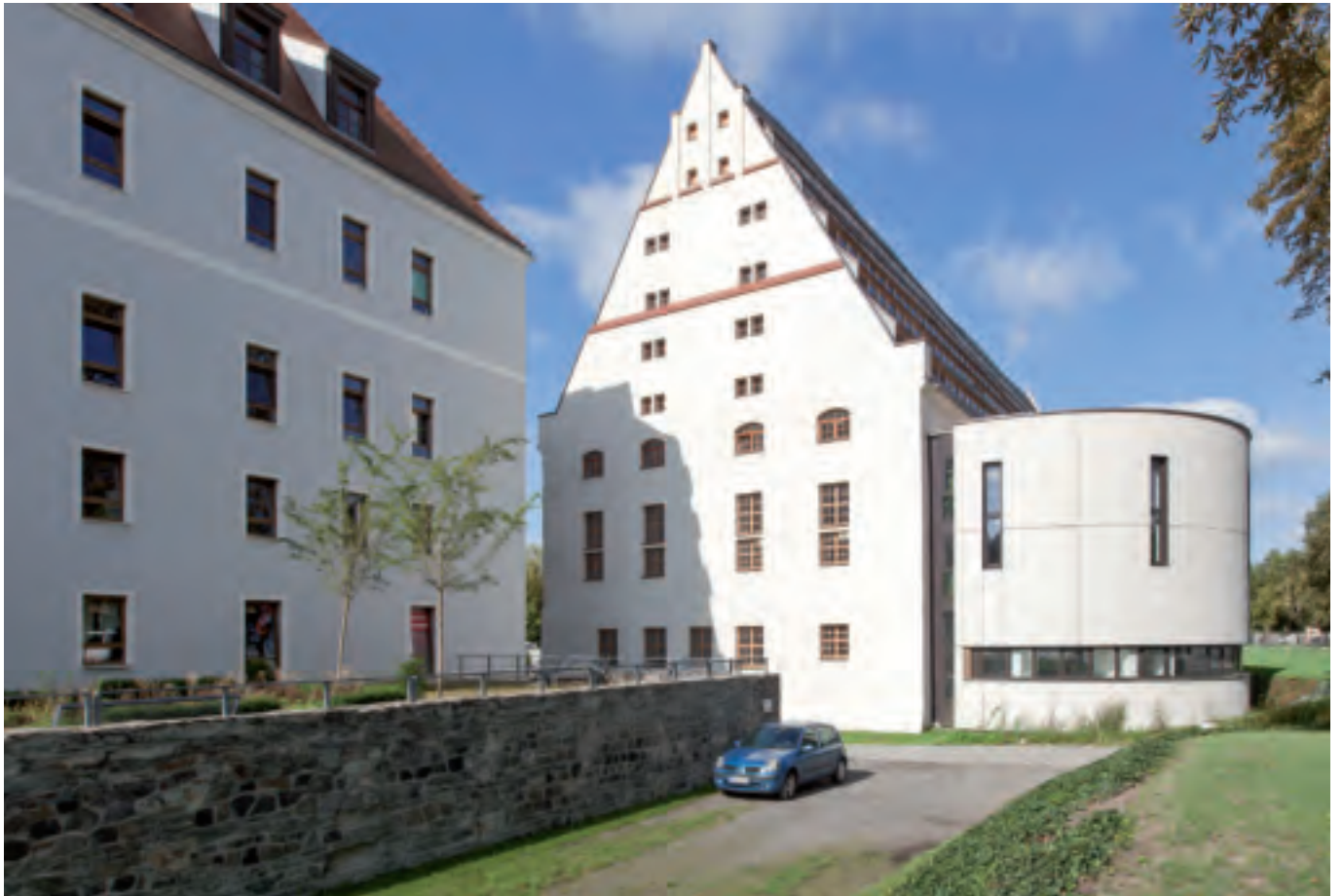
Gabel of the granary with new construction on top of the floor plan of the former cloth maker's bastion
