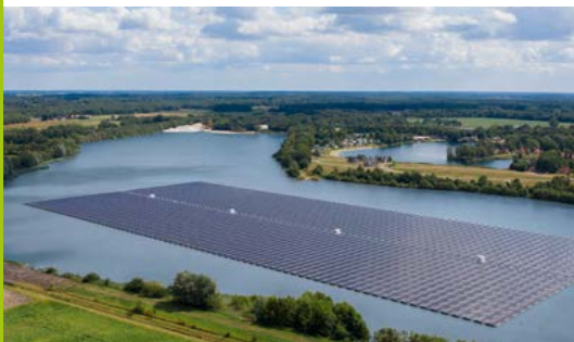
Floating-PV-Anlage in Tynaarlo.
