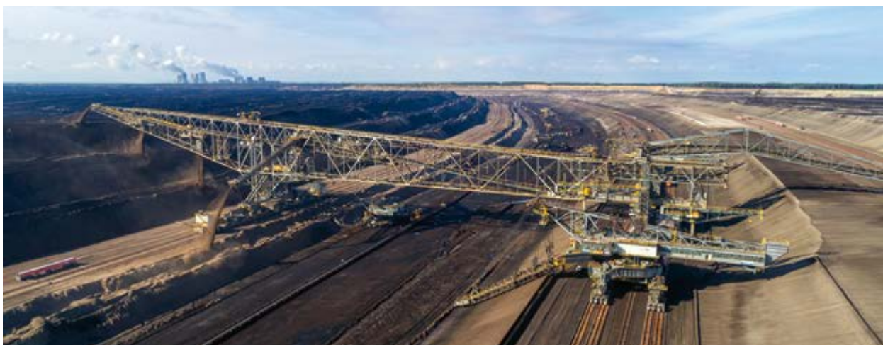
Illustration 3: Opencast mine in Nochten, overburden conveyor gantry F60 (Source: LEAG/Andreas Franke 2018)
