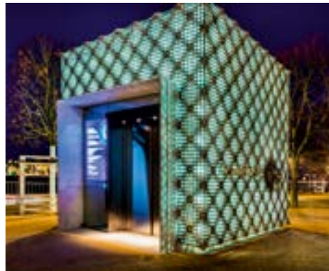
Fully accessible entrance with the elevator on Bruehl's Terrace
